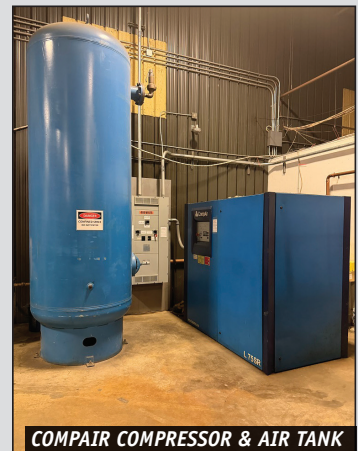
COMPAIR COMPRESSOR & AIR TANK
