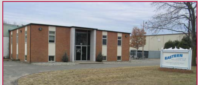
VIEW OF OFFICE BUILDING
