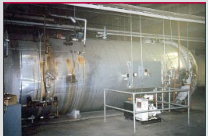
AUTOCLAVE 17' x 8' DIAMETER (SIDE VIEW)
